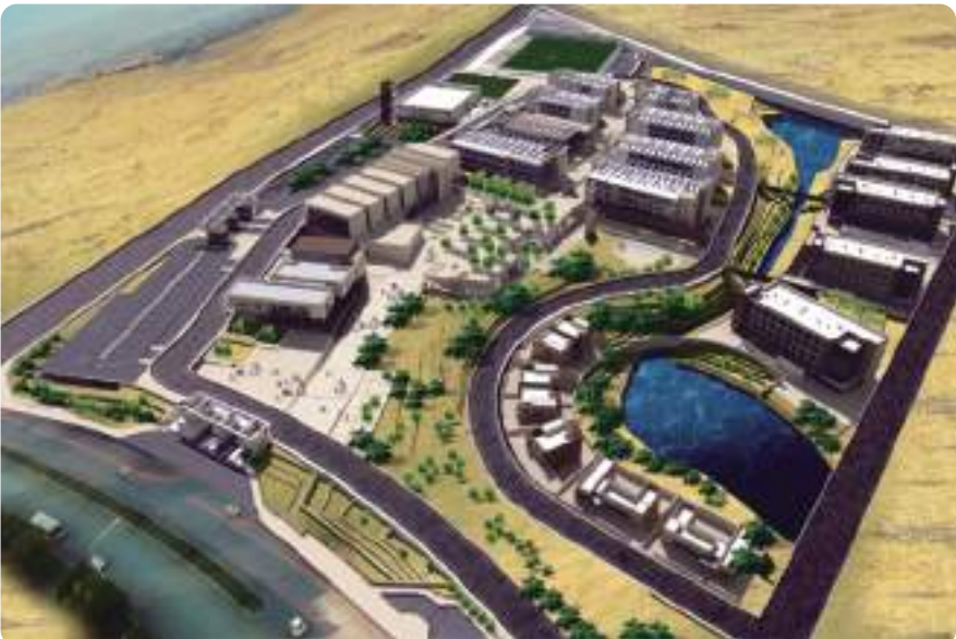
Komar University Country: Iraq City: Sulaymaniyah Outdoor Units: Air-cooled screw & scroll chiller Indoor Units: FCU & AHU Total Capacity: 2,350kW
