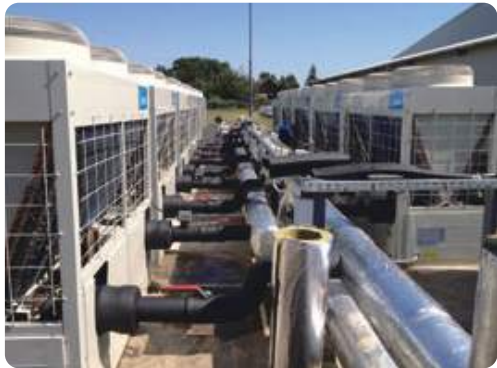
KUKA Robotics in Hungary Country: Hungary City: Füzesgyarmat Outdoor Units: Air-cooled scroll chiller Indoor Units: FCU & AHU Total Capacity: 715kW
